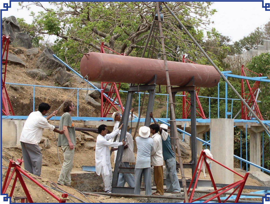
Erection of steam tank, Gyan Sarovar
