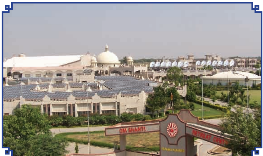
200 kwp solar power plant at Om Shanti Retreat centre near New Dehli, 2006
